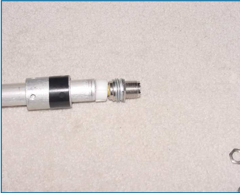
Figure 3 - Next insert the dielectric material saved when the cable was prepared.
